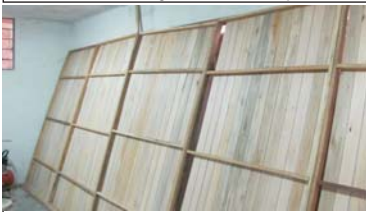
There are 370 tongue and groove boards in a pre-fab house
