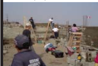
Spirit & Truth Team on construction site in Patacutec
