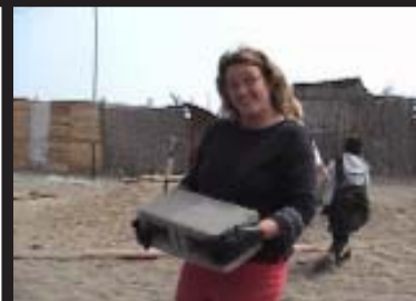
Anne moving block on the construction site in Patacutec
